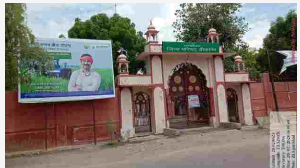
Hoarding Installation_ Jila Parishad
